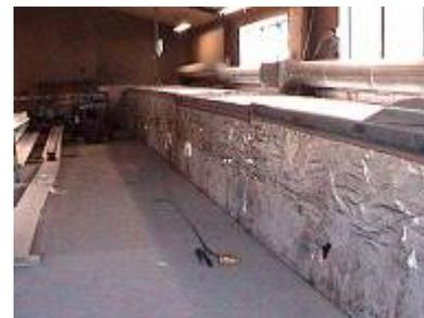
(b) Using insulated covers and gas-fired heating for curing the beams
