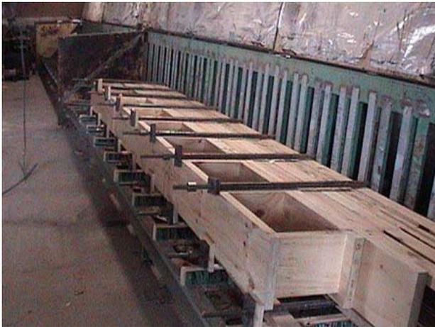
(a) Fabrication of long span Boxed beam
