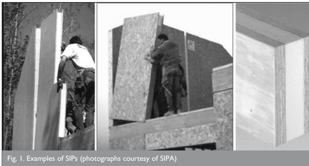
Fig. 1. Examples of SIPs (photographs courtesy of SIPA)
