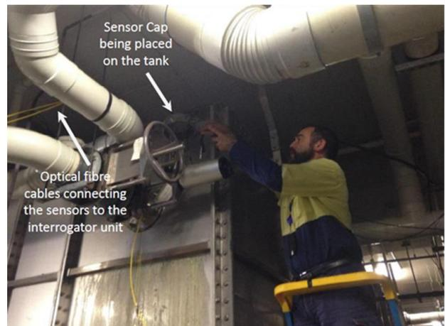
Figure 5: Installation of sensors setup in sewer
