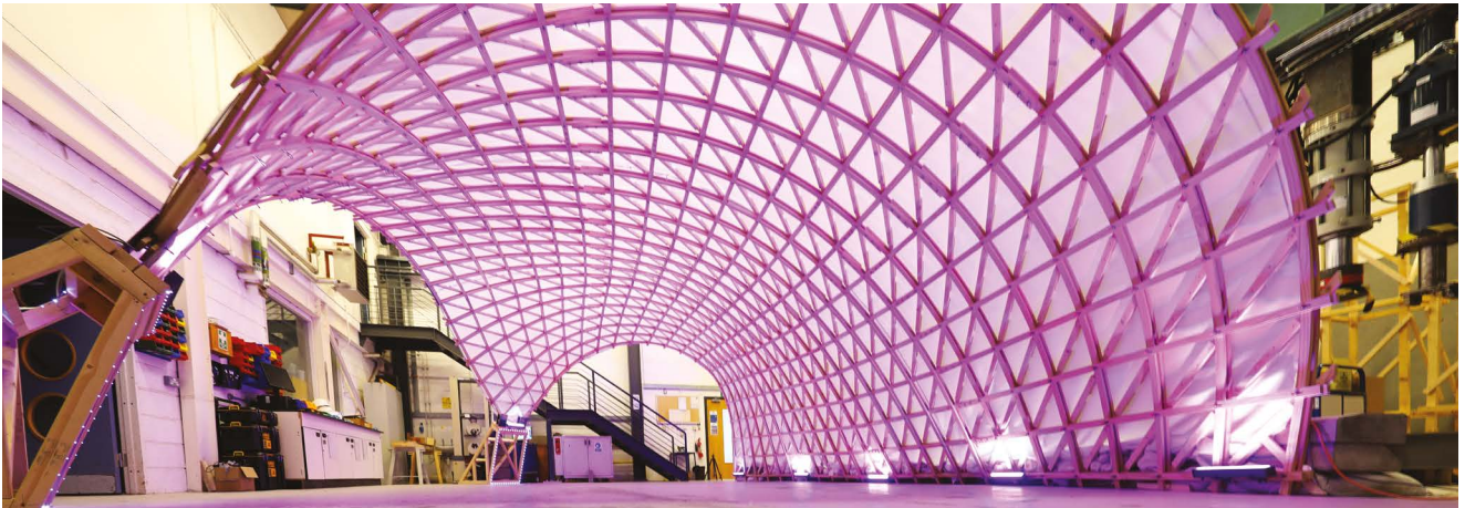
The innovative bamboo-timber composite gridshell
