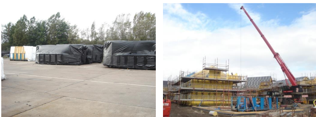
FIGURE 2.9 Panels wrapped in impermeable materials awaiting transportation to the construction site (left); positioning of the panels by crane, on site (right).
