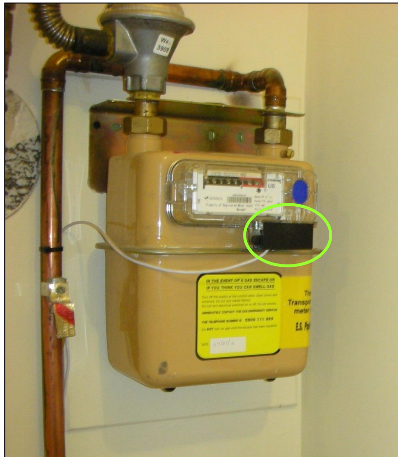
Figure 3.7: Photo of Ewgeco's pulse block (highlighted) connected to a pulsed enabled 'dumb' gas meter
