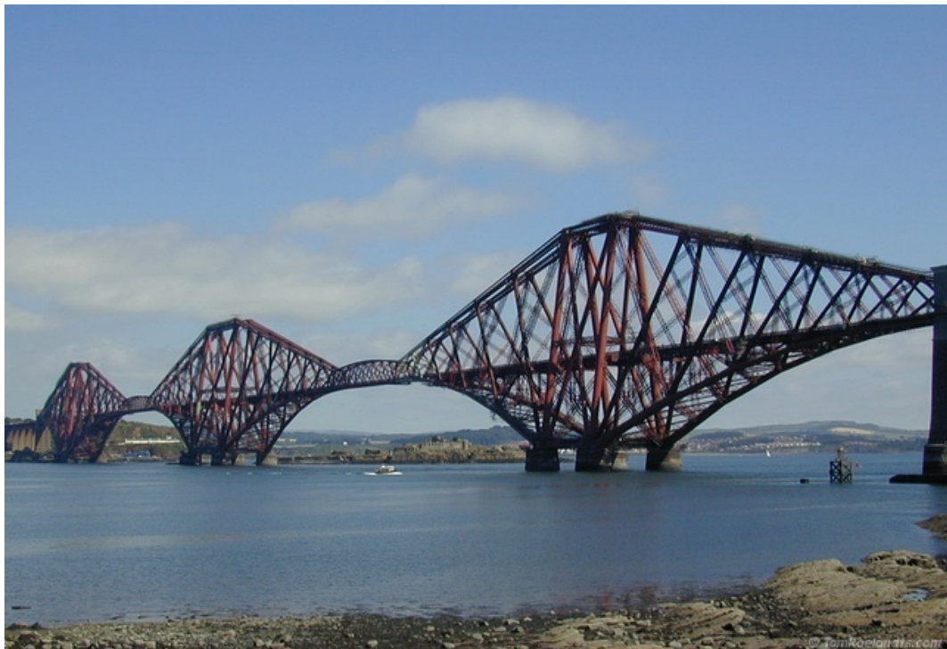
Figure 1.1.2 – Forth Railway Bridge (Roelandts, n.d.)
