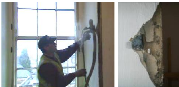
Figure 5. Pressurised expanded polystyrene bead insulation in walls
