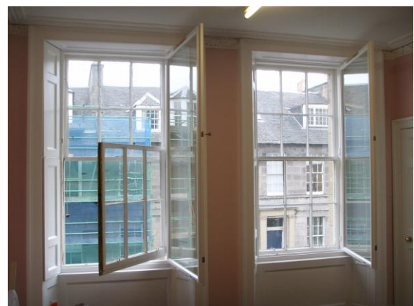
Figure 7. Secondary aluminium windows behind existing sash & case timber windows
