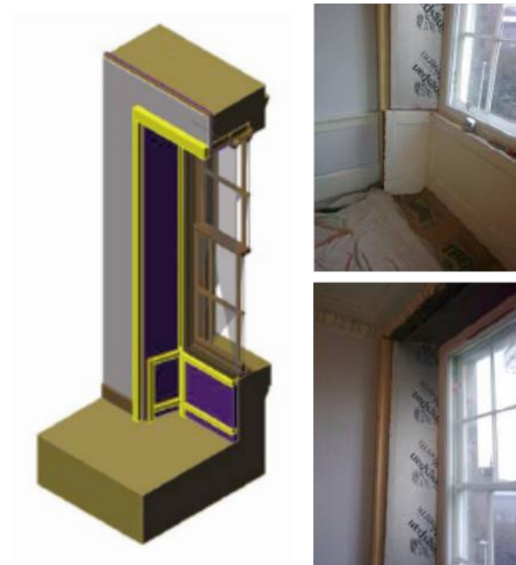
Figure 6. Rigid insulation on the reveals and under windows
