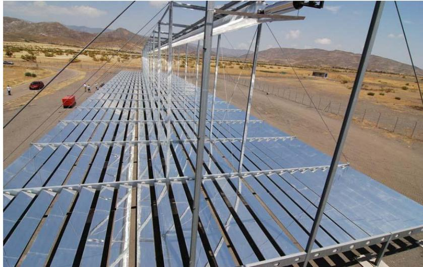
**Figure 2.13** The MAN linear Fresnel demo collector erected on the Plataforma Solar de Almería (PSA) [26]
