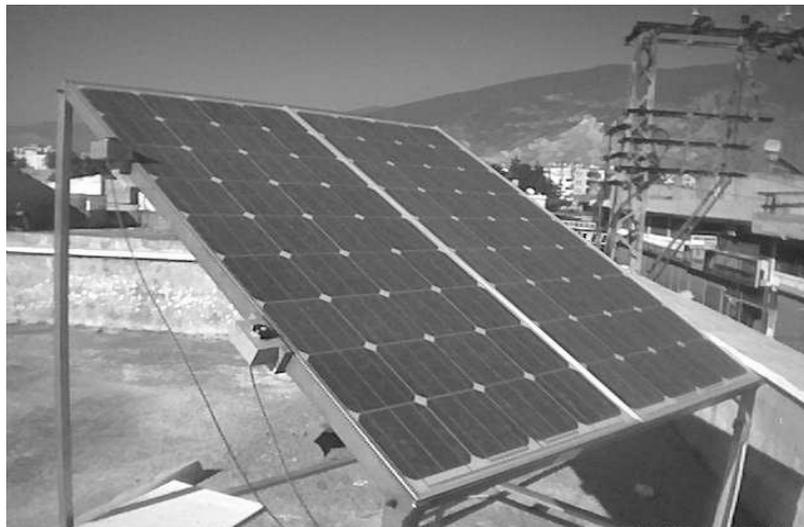
**Figure 6.10** Photovoltaic modules mounted at an angle of 36° situated on the top of a building in Iskenderun, Turkey
