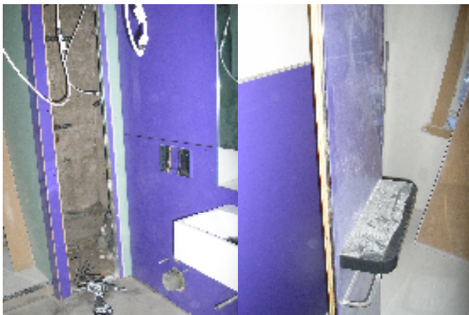
Figure 4: Pre-finished 'kit' panels being installed on site. (Courtesy: Sir Robert McAlpine)
