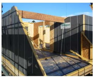
Figure 1: Timber platform frame during construction
