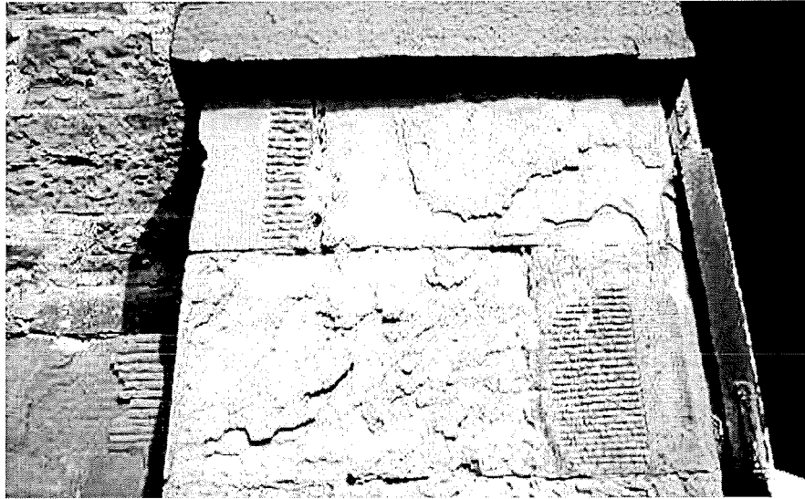
Fig. 3.7 – Stone wall showing spalling
