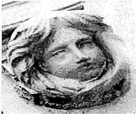
Fig. 4.5 – Eventual erosion of stone from cleaning
