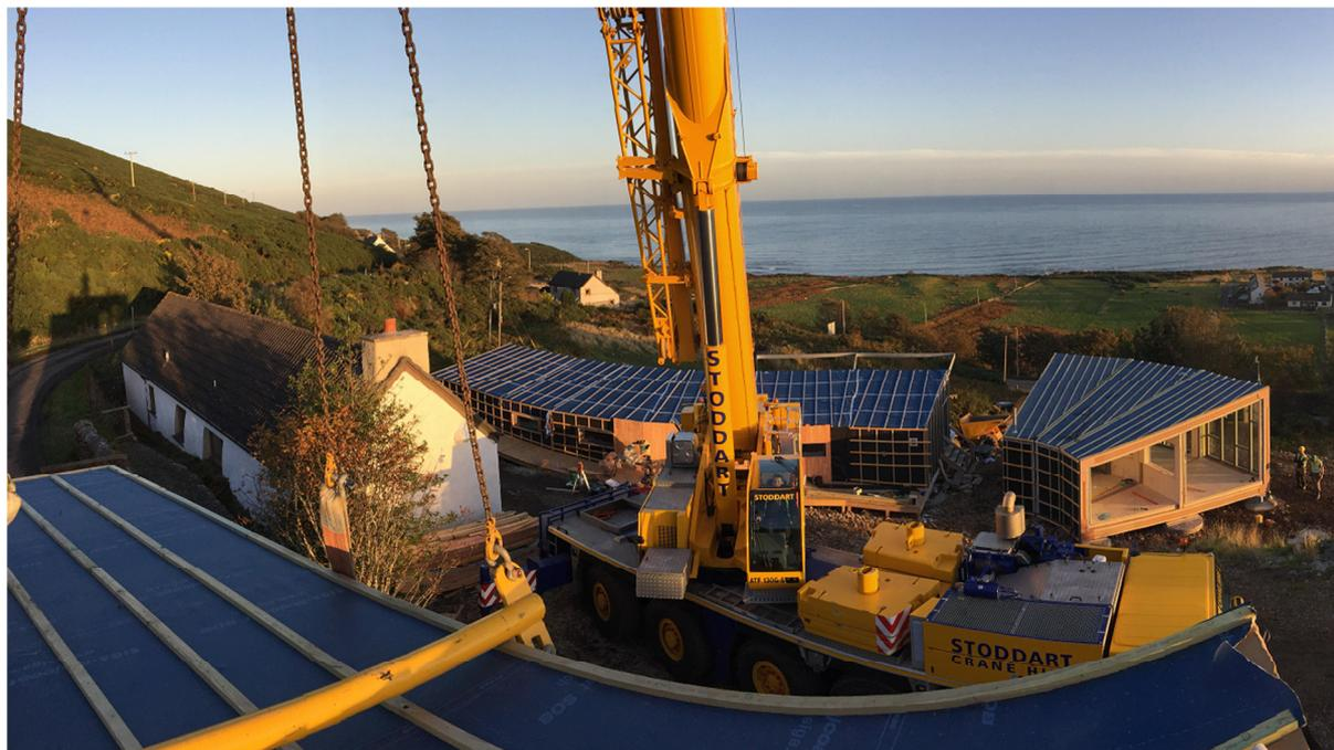
Developments in offsite manufacture and modern methods of construction (MMC) mean that there is far more to offsite timber systems than conventional timber frame construction – such as solid laminate timber products including mechanical laminated systems (nail-lam or dowel-lam also known as Brettstapel); and bonded laminated systems including GluLam and cross-laminated timber (known as CrossLam, or CLT).
