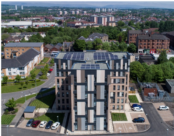
Figure 5: Yoker project in context. Courtesy of CCG.
