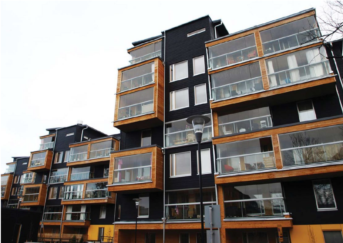
Fig. 8. Seven-storey volumetric timber apartment block buildings in EU. Photograph(s) taken by: Duncheva, T.
