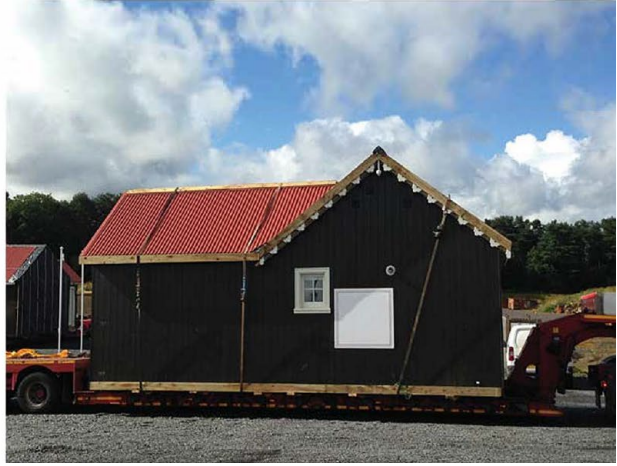
Fig. 5. Examples of different transport methods for offsite timber panels and a volumetric module, whose height necessitates the use of an articulated trailer: (a) Standard trailer with stacked open timber panels; and (b) Articulated trailer with a volumetric timber module. Photograph(s) taken by: Duncheva, T.
