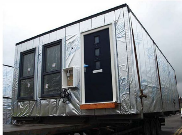
Fig. 1. Examples of offsite timber systems studied in this paper: (a) Closed timber panels; and (b) Volumetric timber module. Photograph(s) taken by: Duncheva, T.
