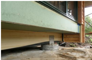
Figure 19 - Accoya® Glulam in-situ
