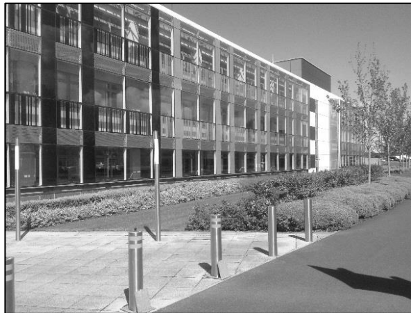
2 (b) South facing façade
